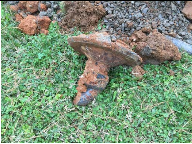
Photo 7 – TP-3 – Pipe connection encountered in test pit
