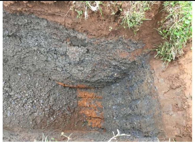
Photo 20 – TP-11 – Apparent CR6 material underlain by natural soils
