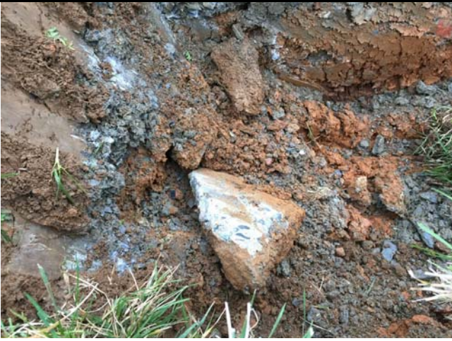
Photo 13 – TP-7 – Concrete material encountered in test pit
