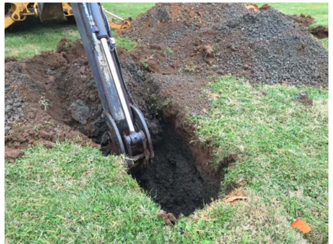
Photo 18 – TP-11 – Excavation of test pit
