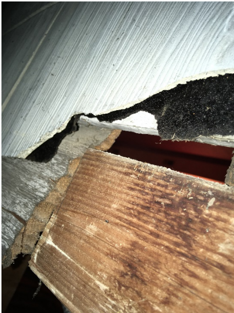
Gray Transite siding on Exterior Theater Walls
