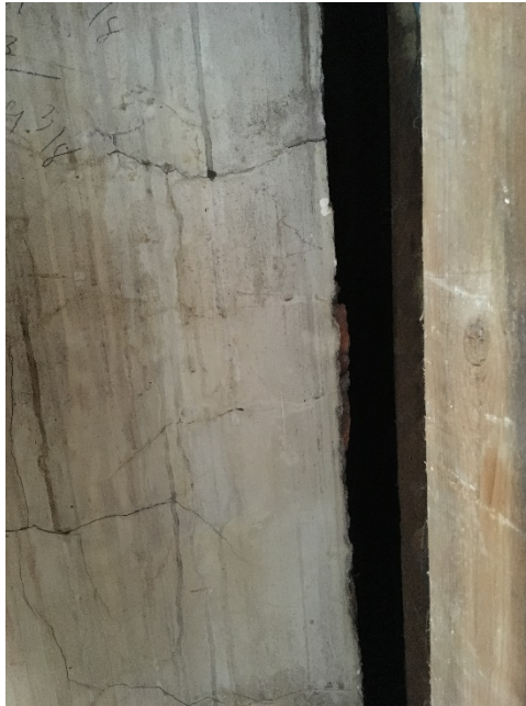
Gray plaster on Chimney as seen from 3 rd floor
